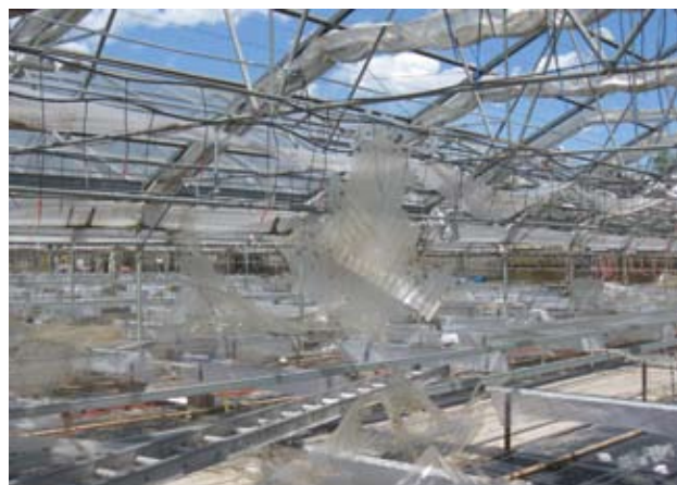
Hail can cause extensive damage to greenhouse coverings. It is essential to protect the crops when they become exposed to the elements after the loss of the roof.
