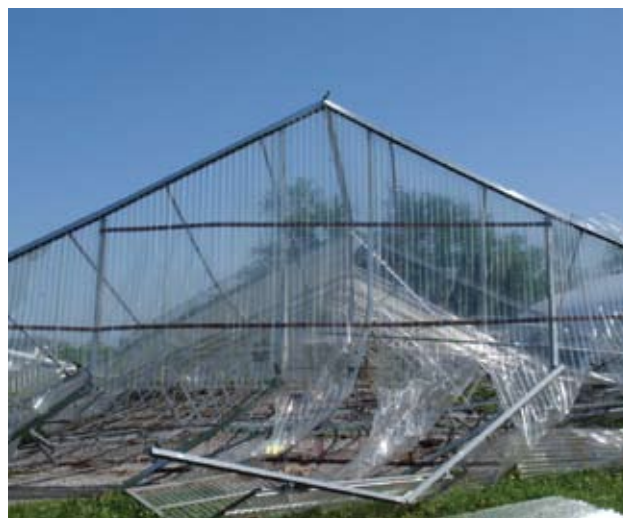
Greenhouse structures can be designed to withstand winds up to 100 miles an hour with minimal to moderate damage.
